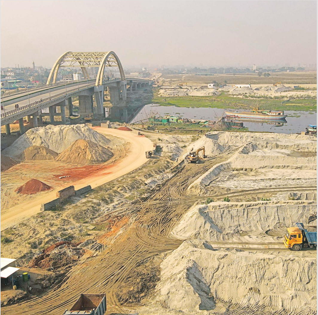
Sand filling in the Boro Beraid, Dhaka © Rakib Hasan, 2024
