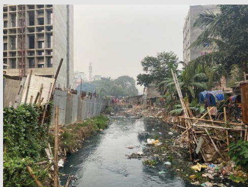
Figure 3.20: Sec 6 Digun Khal Encroached by Floating Houses.
