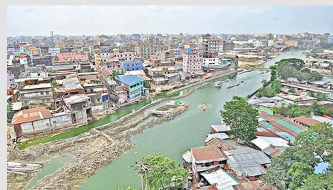
Figure 5.12: Multi-storied buildings and various structures have been built by occupying the Rajakhali canal in Chattogram even though no construction is allowed within 12 feet of the canal
