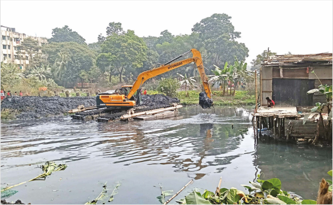
Waste removal from Baunia canal, Dhaka © Md Jahidul Islam, TBS, February 2025
