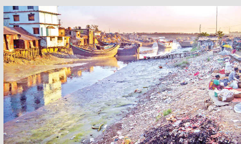
Figure: 5.11: The photo shows a huge amount of silt deposited in the Chaktai Khal, one of the main canals which drains out rain water from the port city, is creating hindrance to smooth flow of water
