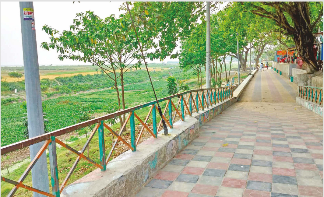
Restoration and beautification of Padma river bank, Rajshahi © Sarjil Ahmed Khan, 2023
